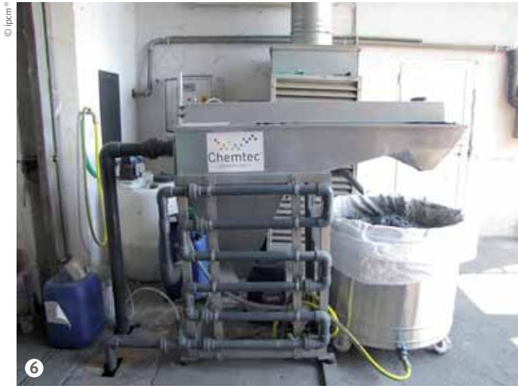
Figure 6: The waste water treatment plant installed by Chemtec.
