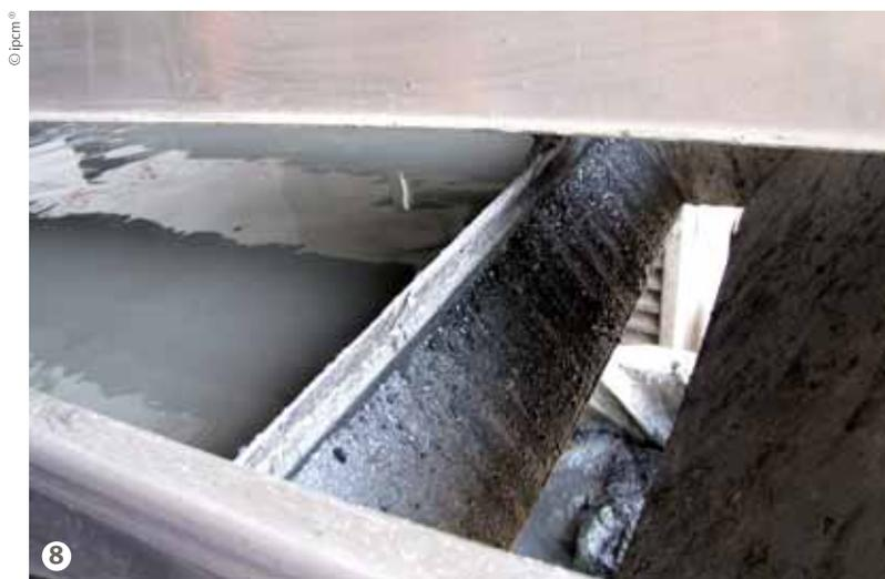
**Figure 8: The scraper collects the inert molecules and pushes them into the sludge container.**
